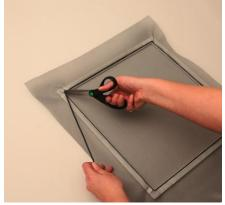
When you reach the end of the 4<sup>th</sup> side cut the spline with a pair of scissors and push the end down into the corner.
